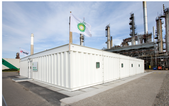
Figure 3 Prefabricated blast building with corrugated steel walls by Hertel/InterDam.
