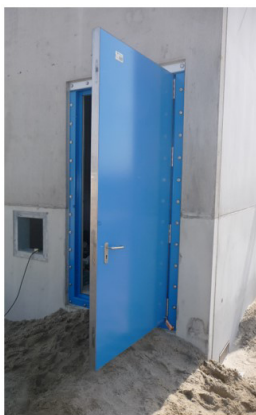
Figure 1 Precast concrete building, LNG Terminal Botlek
