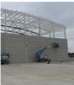
Figure 2 Concrete Firewall | Precast Blast Walls | Precast Concrete Walls Panels | ACP (Concrete) Ltd (thomasarmstrongacpconcrete.co.uk).
