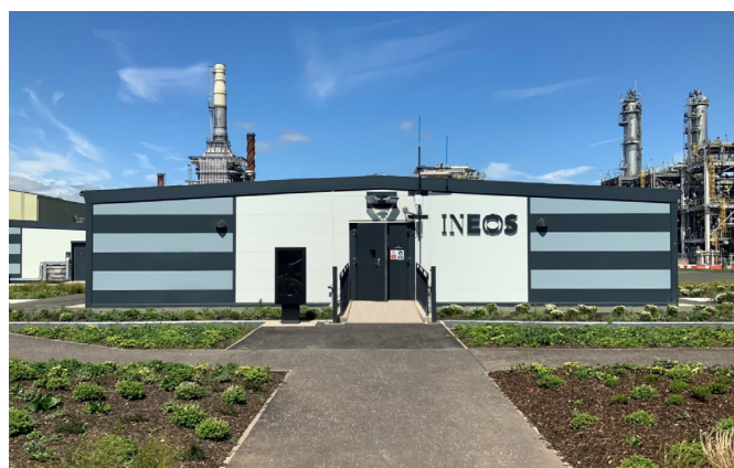
Figure 4 Ineos control building with steel fire- and blast resistant sandwich panels.
