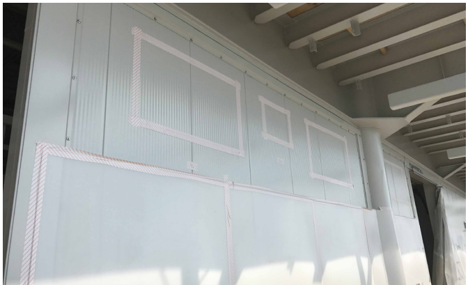
Figure 13 Generation IV internal sandwich panel wall A60 with protection board up to 8 feet and markings (top of wall) for 3 square penetrations.
