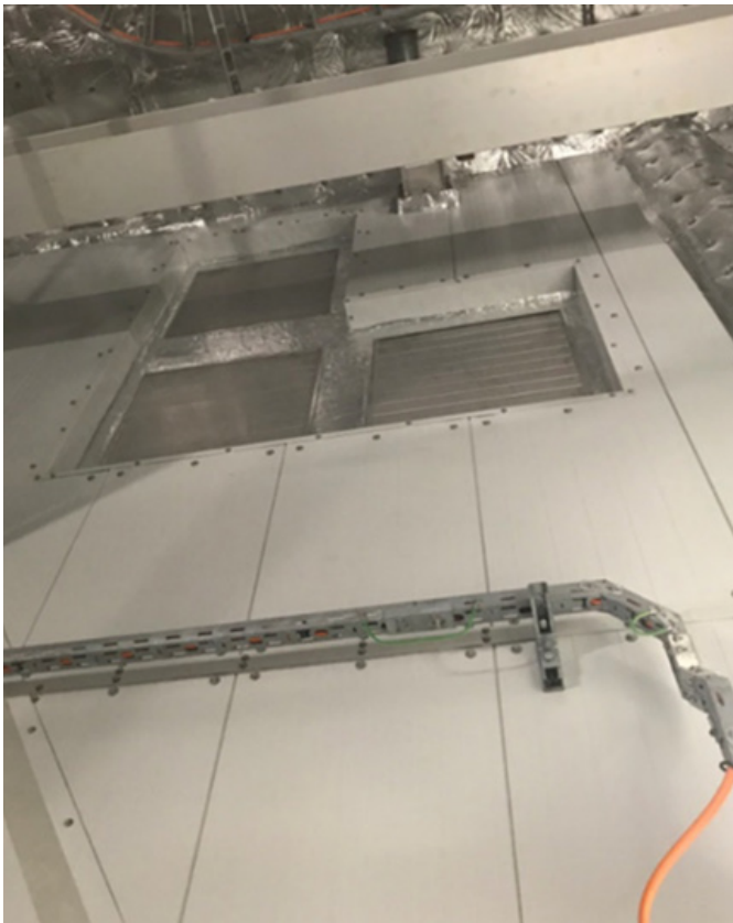
Figure 11 A60 removable panel in Generation IV external sandwich panel wall, seen from outside.
