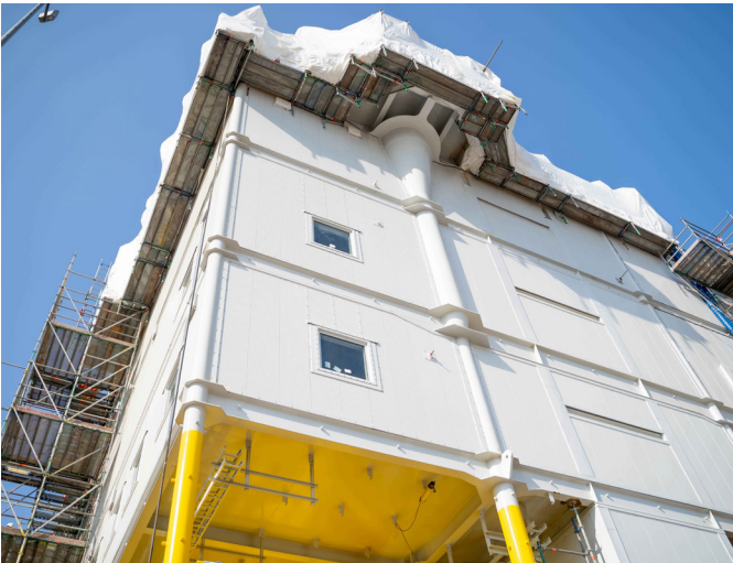
Figure 3 Generation IV external sandwich wall panels on OSS substation including 2 windows.
