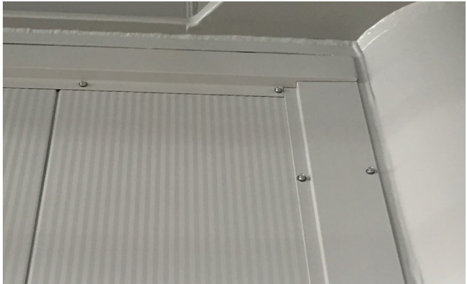
Figure 17 Top and side detail of Generation IV sandwich panel wall system including screwed on flashings. Seen from inside.
