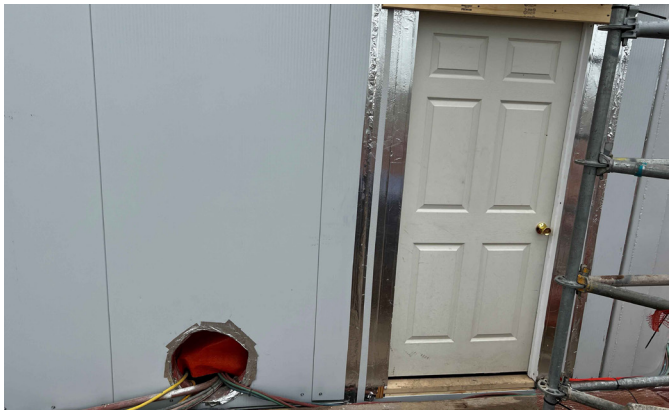
Figure 12 Temporary wooden door in Generation IV external wall (combination is not fire rated yet, but can be closed off and handed over as clean room in the construction phase of the substation).
