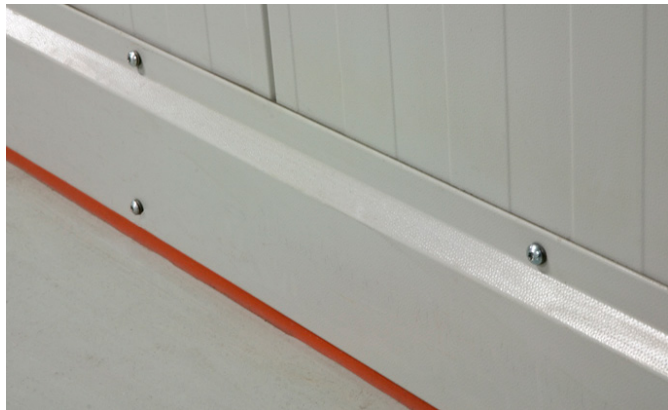
Figure 16 Bottom detail Generation IV sandwich panel wall system including screwed on flashing. Seen from inside.
