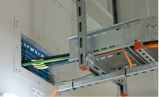
Figure 6 Cable penetration detail of Generation IV sandwich panel wall system. Seen from inside.
