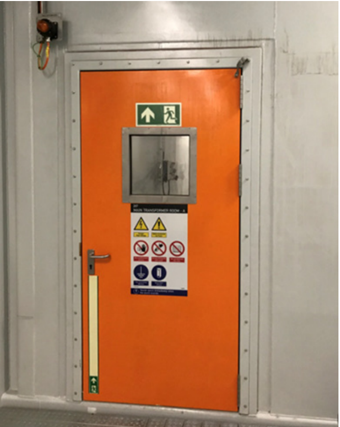
Figure 4 Double sealed hinged door including vision panel and panic bar inside, built into a Generation V wall, welded stressed skin outside and bolted sandwich panels on the inside.
