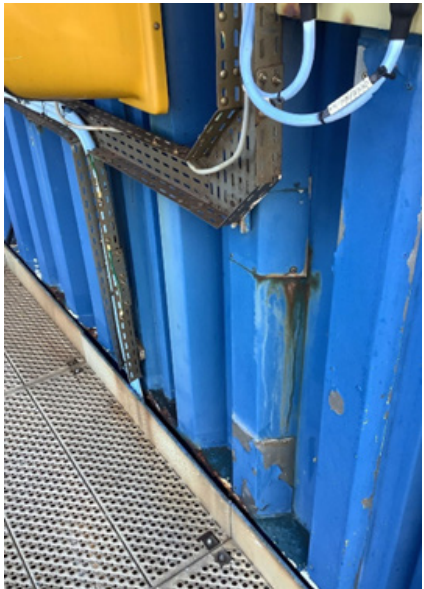
Figure 1 25 years old, patched up offshore fire and blast wall Generation II.
