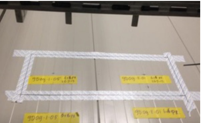
Figure 5 After clean room handover Electrical supplier can exactly note the location of the penetration in the already installed Generation IV sandwich panels.
