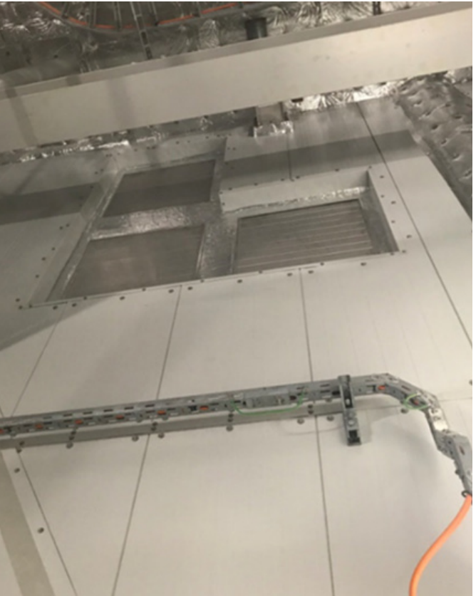
Figure 9 Generation V wall overpressure release vents and bolted on cables on sandwich panels, seen from inside.
