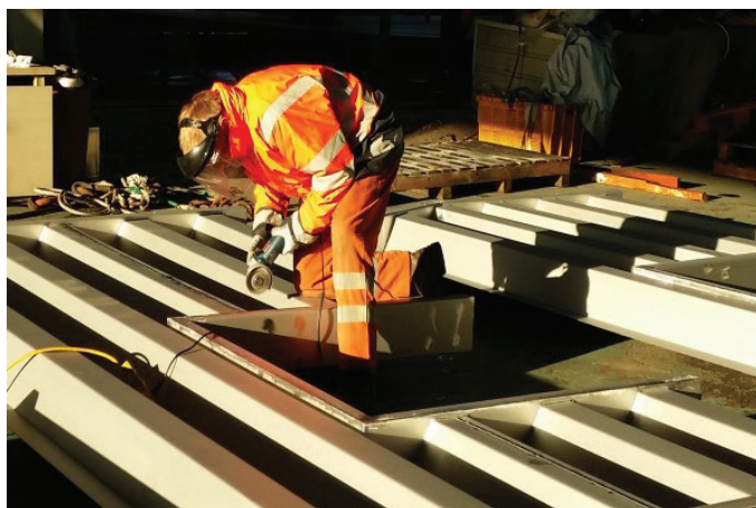
Figure 37: Type II welded wall, pre installation of penetrations required
