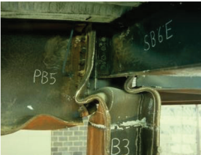
Figure 12: Column head (failure at 5000C)
