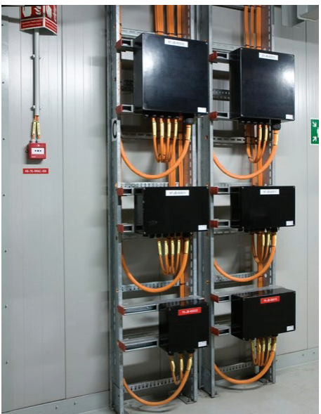
Figure 45: H120 G21 Firewall including supports for electrical equipment
