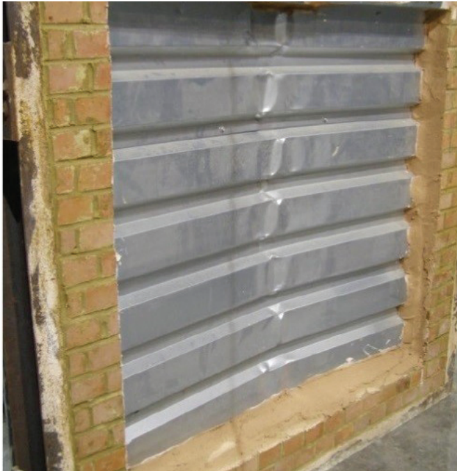
Figure 24: Type III wall exposed side after 1.0 bar blast prior to H120 fire
