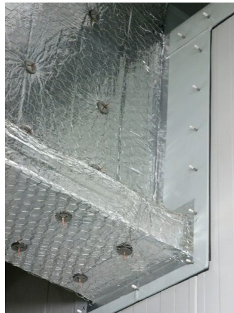
Figure 44: Penetration through H120 rated G21 Fire Panels
