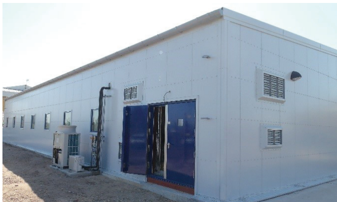
Figure 52: H60 rated G21 Blast panel 0,3 bar blast overpressure including G21 doors and windows. Fire post blast capabilities.
