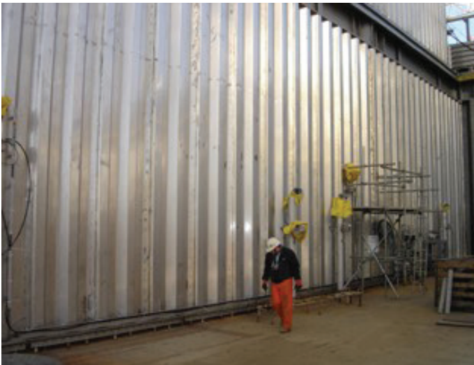
Figure 7: MS Type II walls in use (MS = mild steel)
