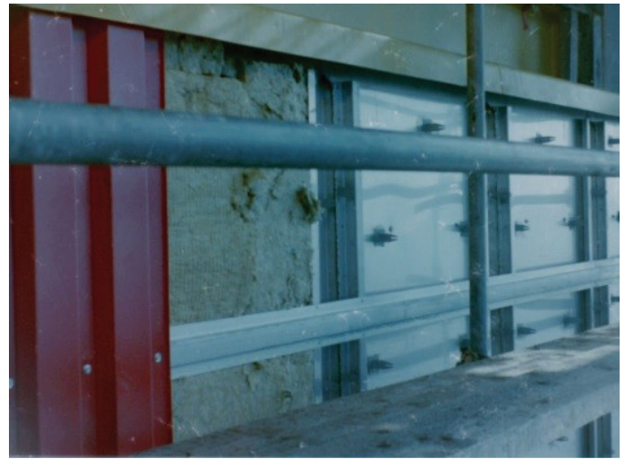
Figure 9: Type III wall under construction
