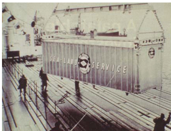
Figure 5: Loading of 1st containers
