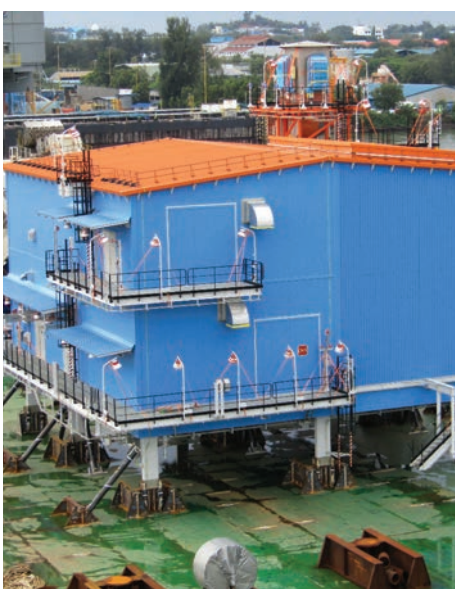
Figure 46: A60 rated G21 panel and bolted removable panel
