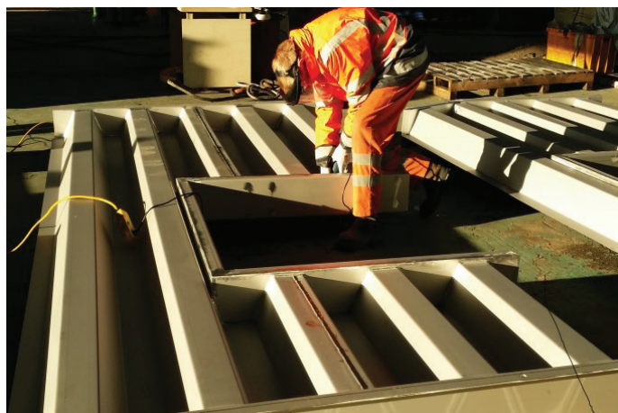
Figure 30: Type II welded wall
