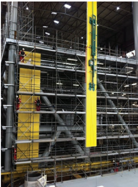
Figure 42: Installation of a G21 Type IV A60 Firewall by crane
