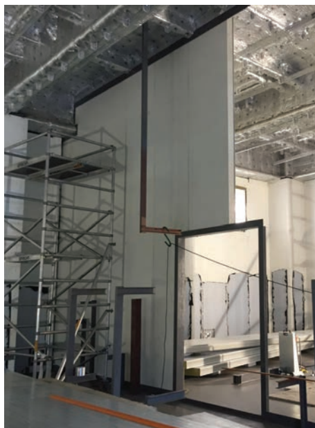
Figure 43: A60 and H60 rated G21 Type IV walls in battery room
