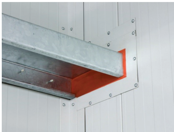
Figure 49: T-junction between external and internal A60 rated G21 FirePanel
