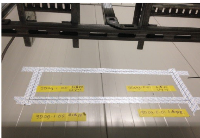
Figure 38: G21 Fire Panel, Type IV bolted wall, installation of penetrations on the spot
