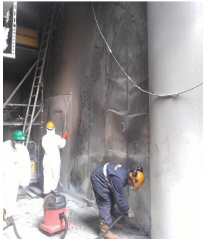
Figure 14: Contained fire on G21 Fire Panel, Type IV A60 sandwich wall (2014)
