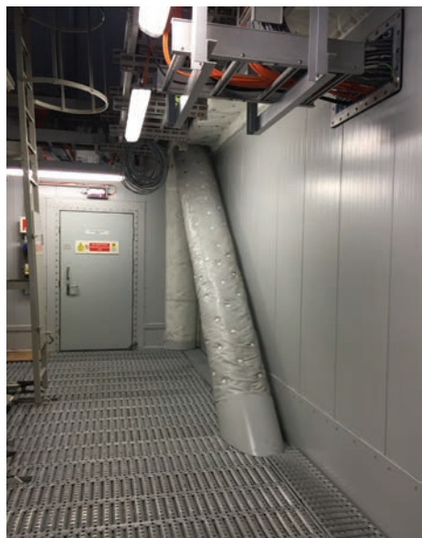
Figure 47: A60 rated G21 FirePanel and A60 single leaf hinged door
