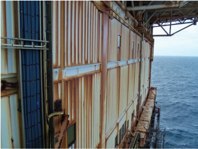
Figure 6: Stainless steel Type II walls during construction
