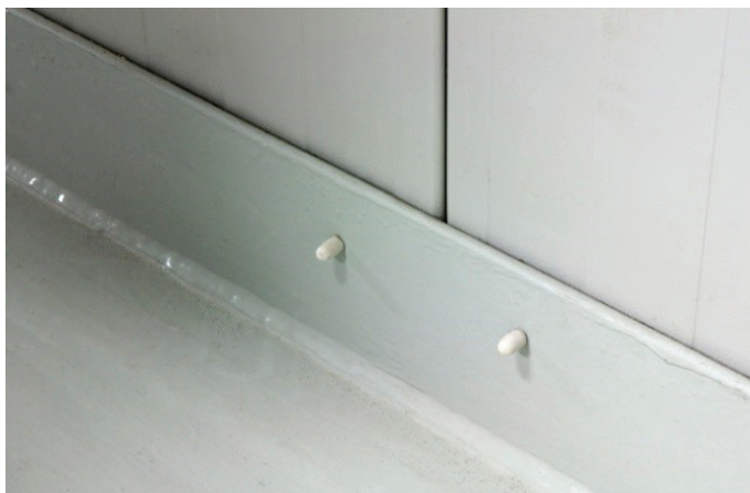
Figure 51: H120 G21 FirePanel / deck connection detail
