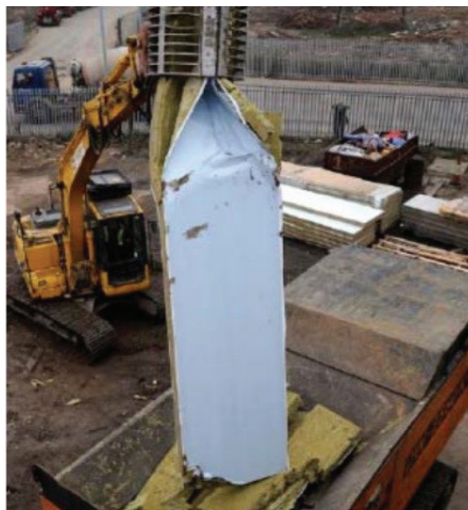
Figure 39: Shredder for obsolete stone wool filled panel
