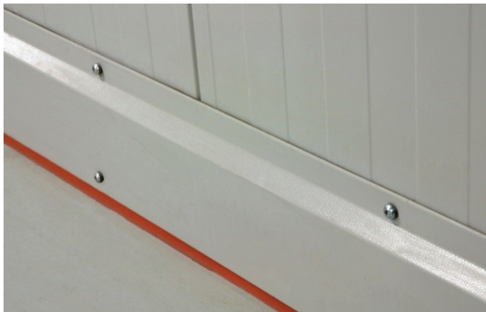
Figure 50: H120 G21 FirePanel / deck connection detail
