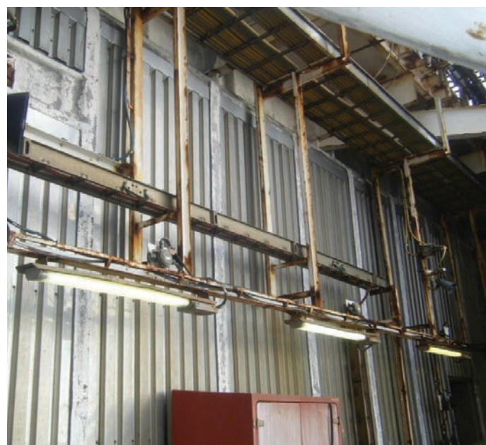
Figure 36: Stainless steel Type III built-up wall exposed for 33 years. Note the difference with the mild steel lighting and walkway supports.
