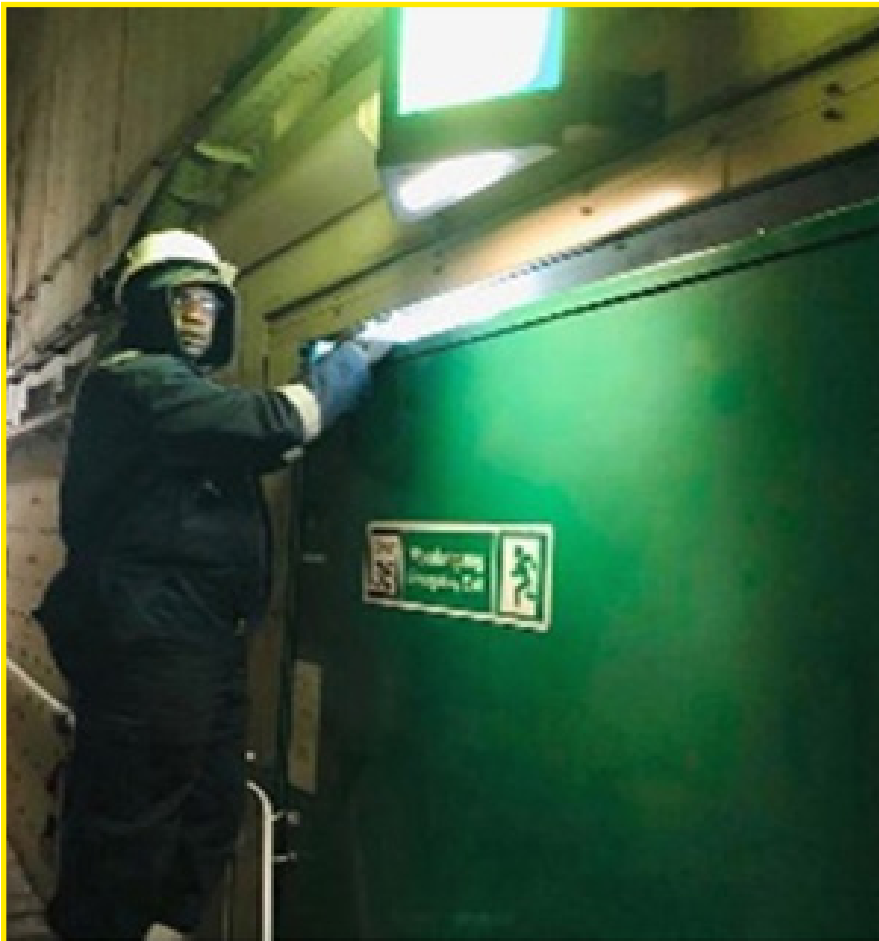
Figure 1: maintenance on tunnel doors should be brought back to an absolute minimum to minimize "tunnel offline", risk and cost.
