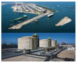
The GATE LNG terminal in Rotterdam port is recently built to unload LNG, store it, and insert it into the European gas grid. High demands were put to the blast- and fire protection of the technical buildings and to the doors InterDam supplied.
