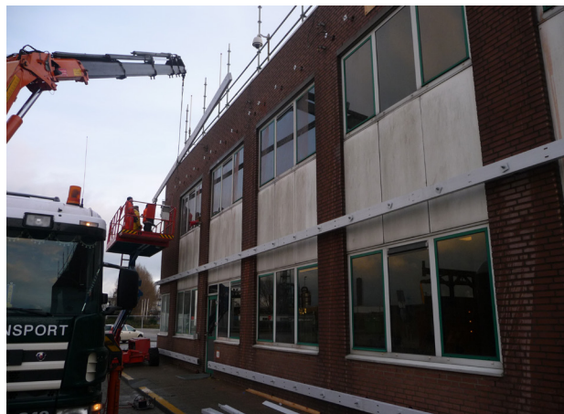
Detail of support structure
