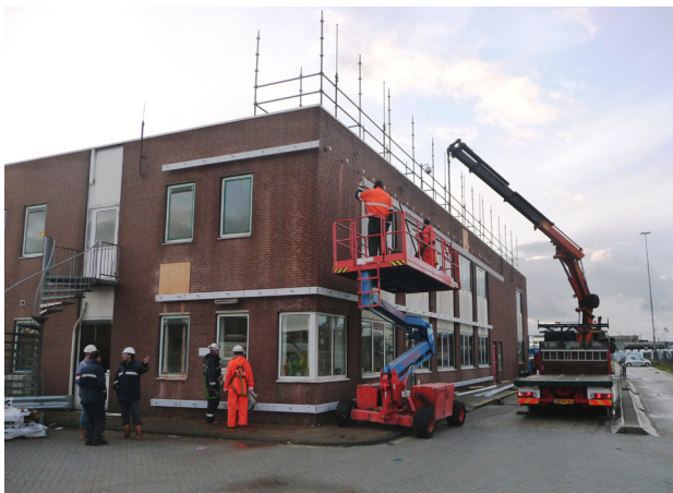
Side view during installation process
