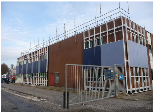
Work under progress: support structure installed and part of blast resistant panels installed
