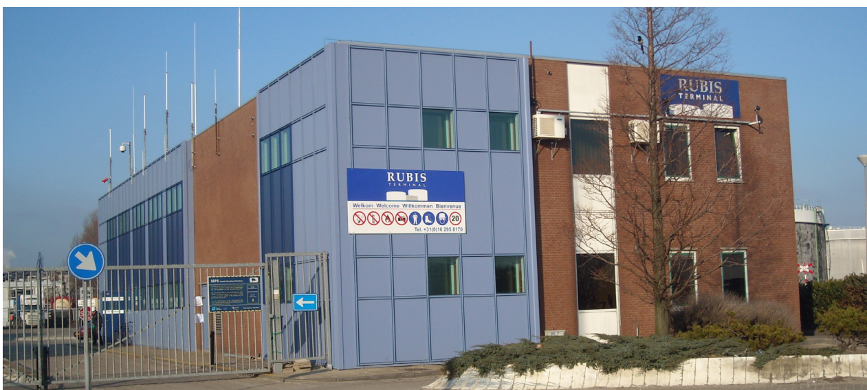
The blast resistant facade completed
